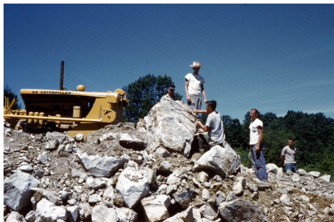
Summer of 1960-placement of revetment riprap and larger stones in the temporary spillway on the south end of the dam
