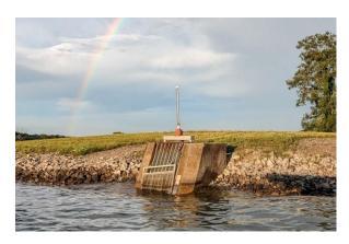
This article on the spillway replacement project will focus on the stilling basin. Our dam is considered a high head, high hazard dam. Head refers to the difference in height from lake level (headwater) to outlet water level (tailwater). According to the DNR the dam is considered high hazard due to the possibility of severe damage and flooding that would occur to the properties downstream of our dam in the event of a failure. The risk of failure is low, but the classification is high hazard.
