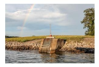
In keeping with the theme of spillway replacement, you may be interested in knowing some of the design considerations. This article will cover the intake structure. The new intake structure takes into account several important factors including: location, elimination of the need for manual gate operation to maintain a consistent lake level, debris protection, and ability to draw the lake down if necessary.
